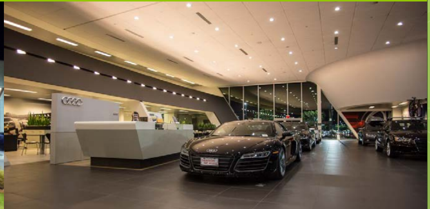
After – 11W LED Can Retrofits
