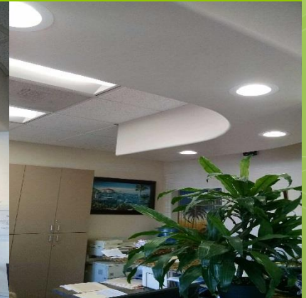
AFTER – 11 Watt LED 5/6" Can Retrofit Kit
