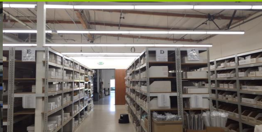
AFTER – 42 Watt LED Strip Retrofit
