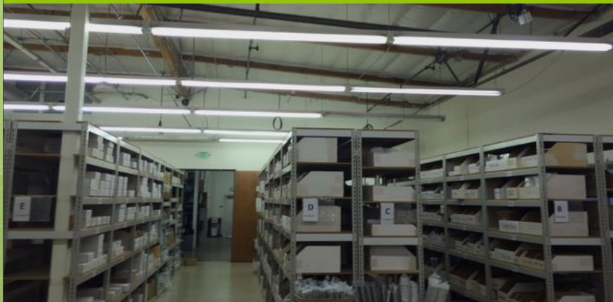
BEFORE – 110 Watt T12 1 Lamp
