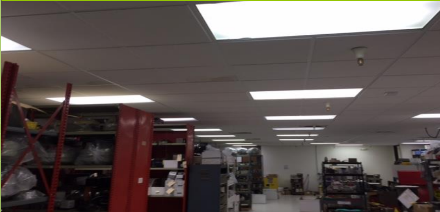
BEFORE – 32 Watt T8 2 Lamp
