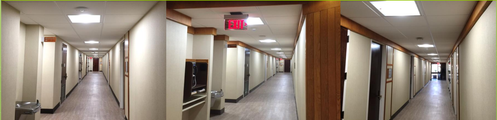
AFTER – 25 Watt LED 2x2 Troffer Retrofit
