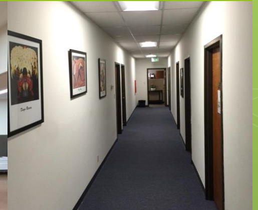
AFTER – 40 Watt LED 2x4 Troffer Retrofit
