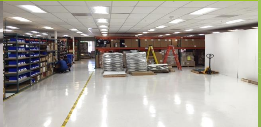
AFTER – 40 Watt Troffer Retrofit
