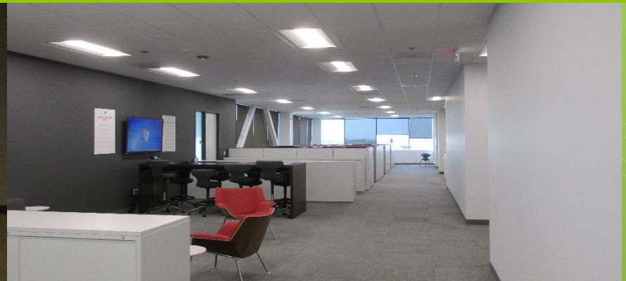
AFTER – 40W LED Troffer Retrofit KUDO
